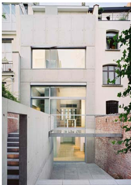
Figure 5e: A cast in situ town house in Brussels, Belgium (Courtesy Architect – Joël Claisse Architectures; Photographer – Jean-Paul Legros, Belgium)
